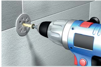
Screwed fixing of insulation boards
