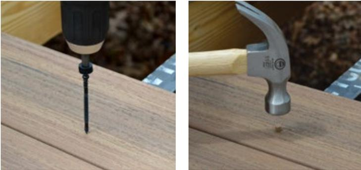
*A special driving tip automatically puts the Cortex® screw at a precise depth. Then, the color-matched plug is tapped in with a hammer.*
