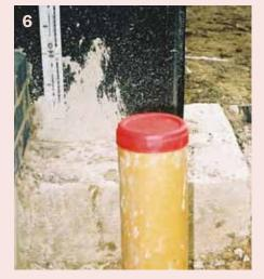
Position the capped section of pipe so that it is about 100mm from the face of the external wall. This will allow space to accommodate a fan if necessary. Provide a plate on the wall to indicate the presence of the radon exhaust pipe.
