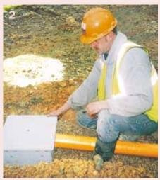
Remove the blanking piece from the proprietary sump and connect a 110mm diameter PVC-U pipe to one outlet of the sump.
