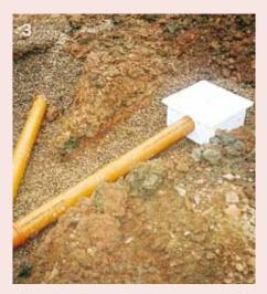
Extend the pipe horizontally so that it passes through the external wall. Ensure that all joints and couplings are airtight.
