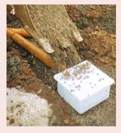
Backfill using a clean permeable material without excessive fines.
