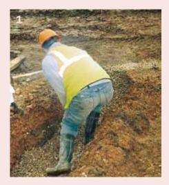
Excavate a pit for the sump, ensuring that, for maximum depressurisation, any fill used beneath the slab does not contain excessive fines.
