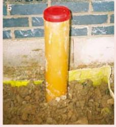
Terminate the pipe just above ground level, and cap it. It will then be ready for extension to form a vent if necessary.
